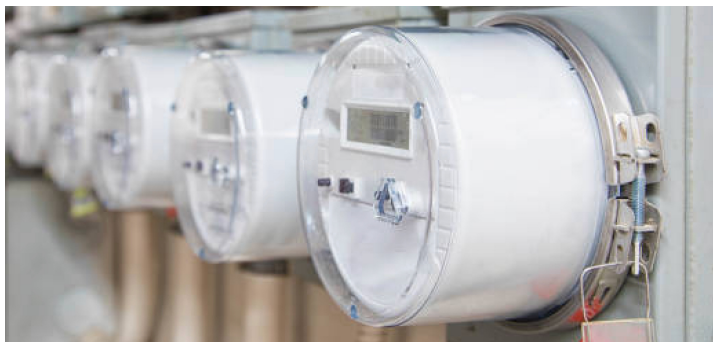
Data Center Power Supply
